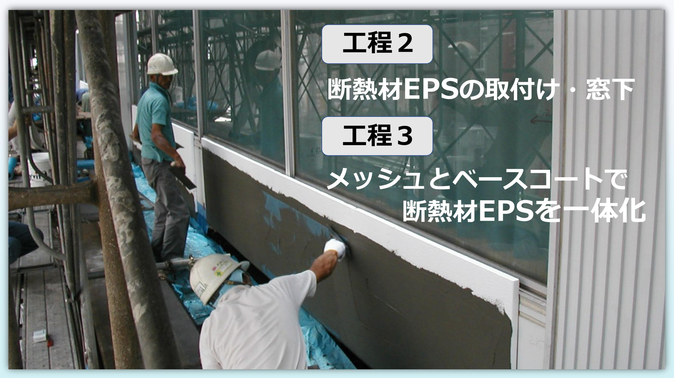
A construction site showing workers on a scaffolding installing EPS insulation under a window. One worker in a white shirt and hard hat is applying a grey mesh to a dark grey base coat on the wall. Another worker in a light blue shirt and hard hat is standing nearby. The window is large and has a metal frame. The scaffolding is made of metal pipes and has a blue safety netting.
